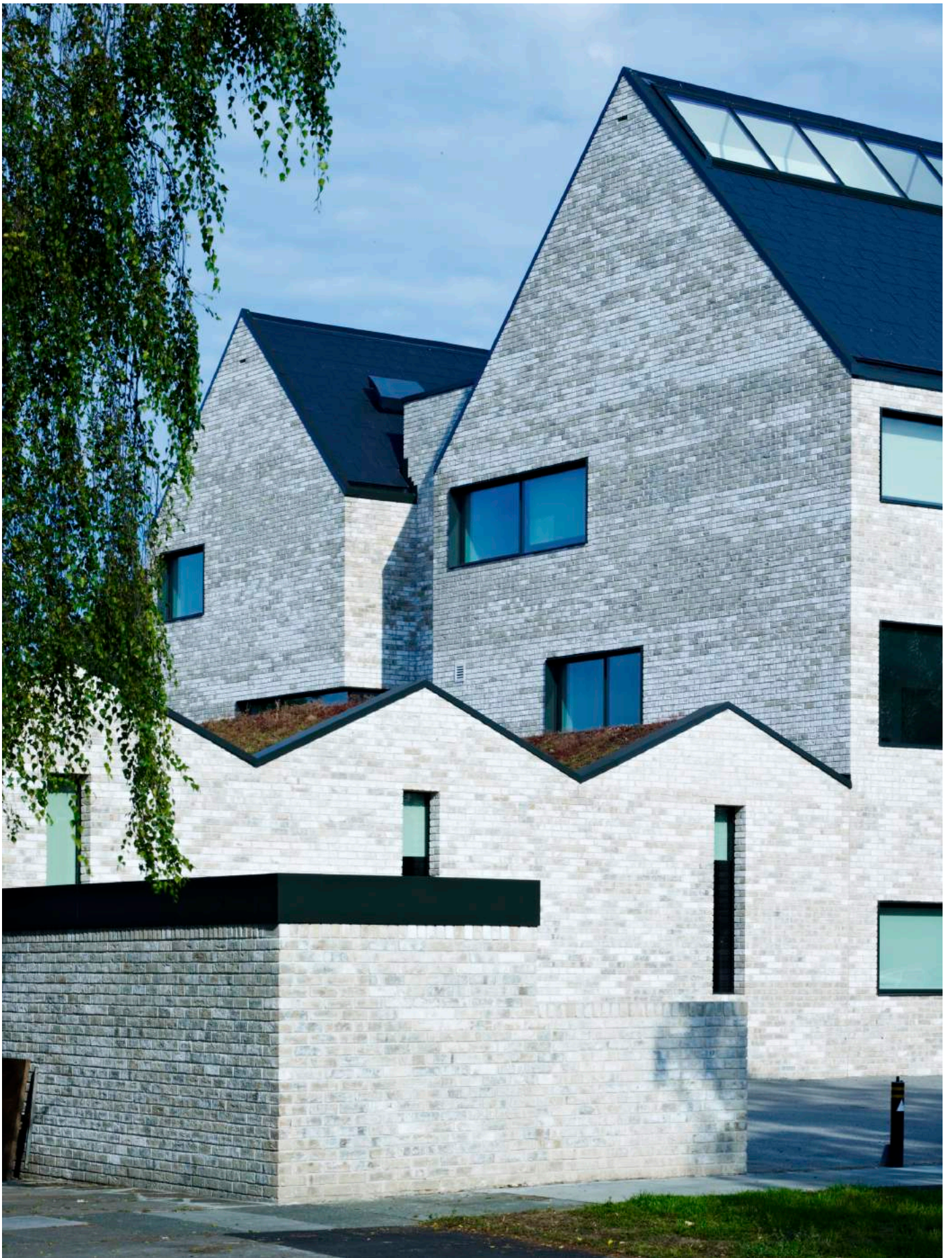
South east corner with rear cables and bin store in forefront
