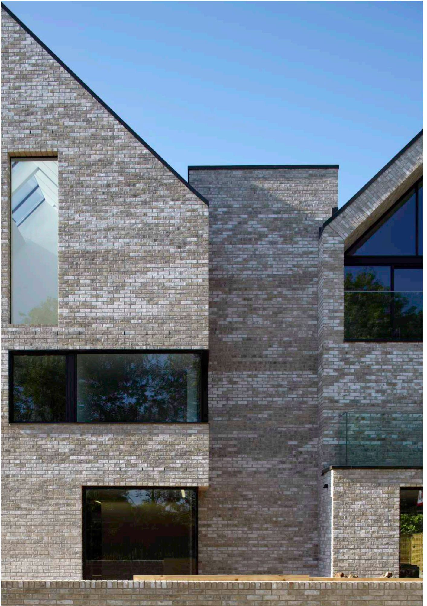
Detail view north elevation: Brick reveals and PPC window trims
