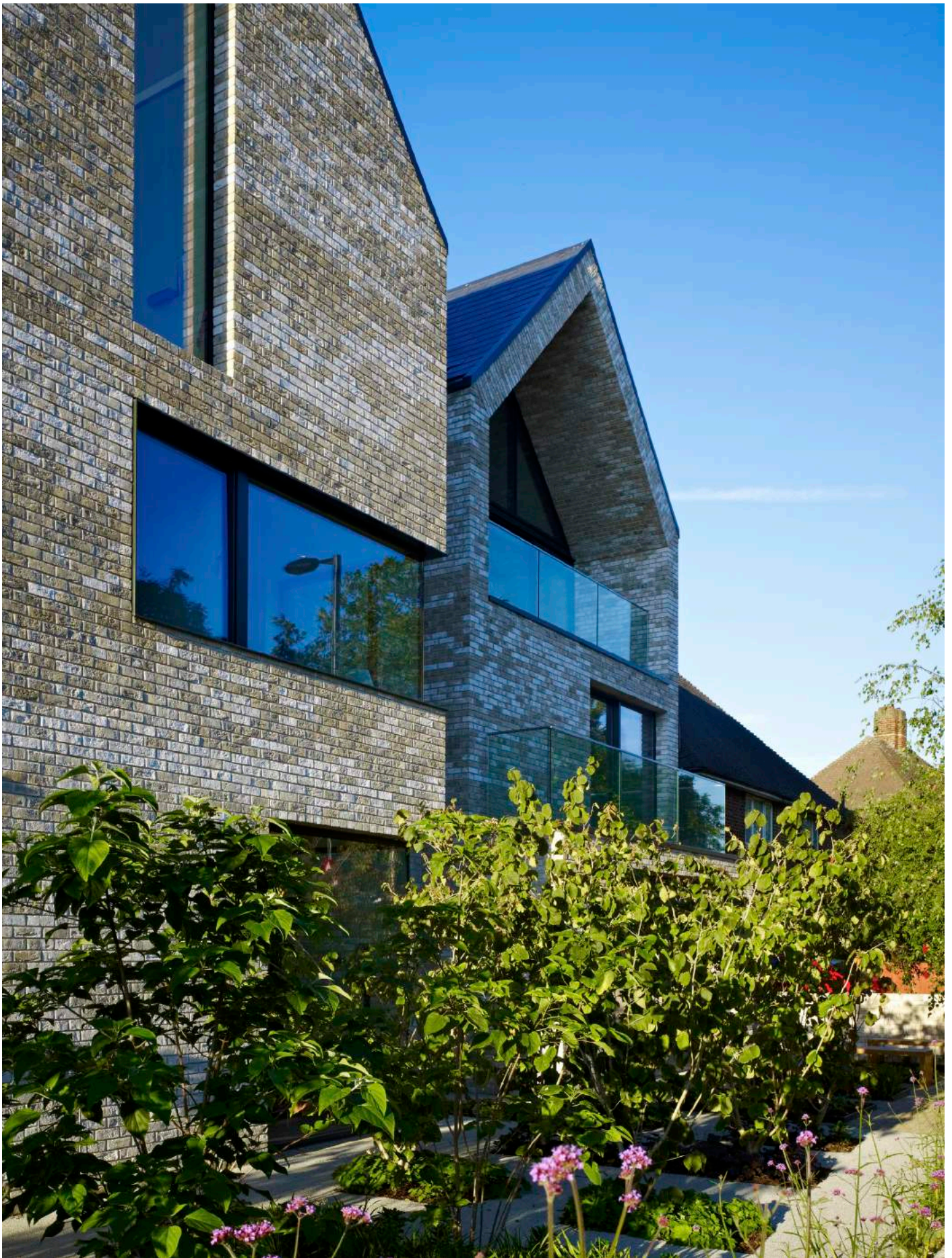
External landscaping along the north elevation
