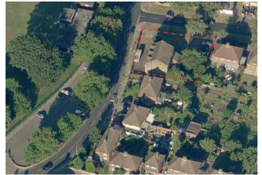
Aerial view looking east towards Barrowell Green
